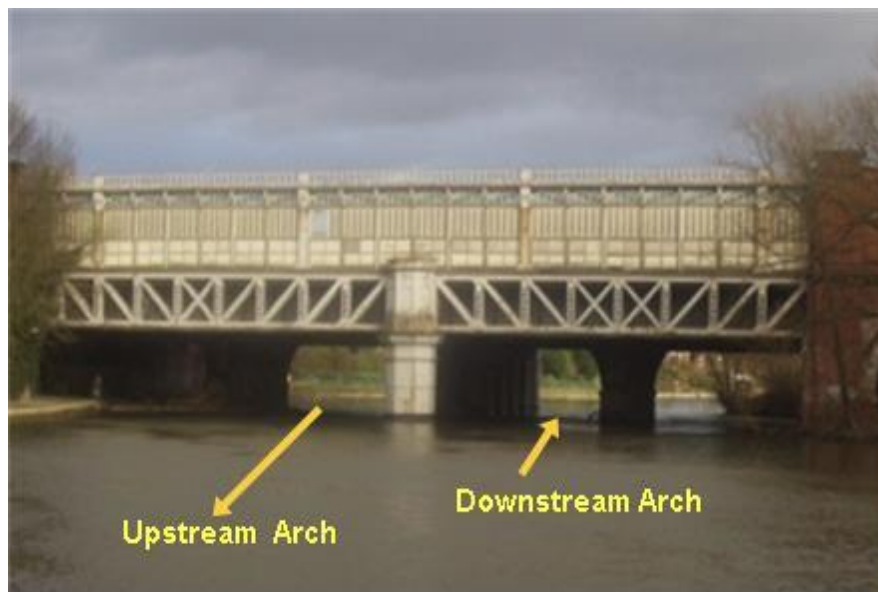
Figure 6 Railway Bridge and Navigable Arches
