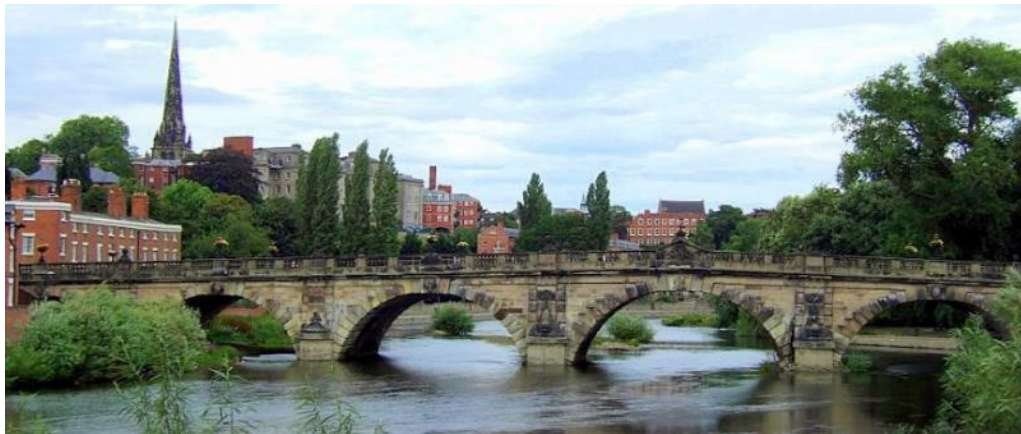
Figure 5 English Bridge Viewed Looking Downstream
